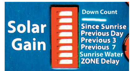
Figure 7: Display of solar gain and setting 2 watering options is controlled by switch shown below.
